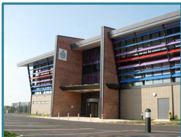
Cumberland BCU HQ – Carlisle
