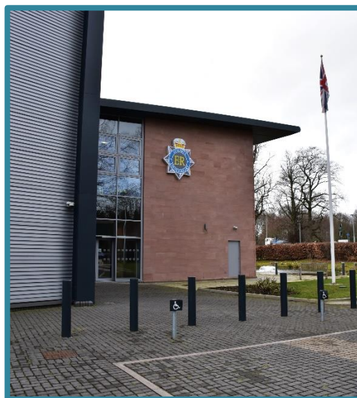
Construction of the Learning and Development Centre was completed in January 2020
