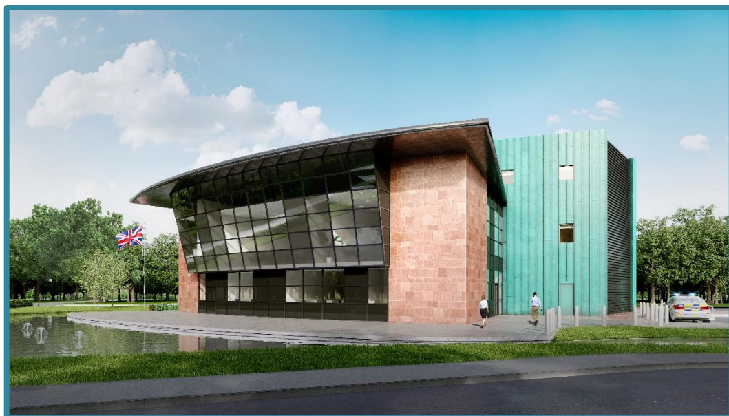
Construction on the Eden Deployment Centre commenced in May 2018 (design image)
