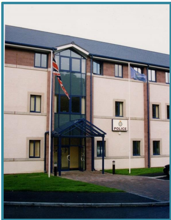
West TPA HQ – Hall Brow, Workington
