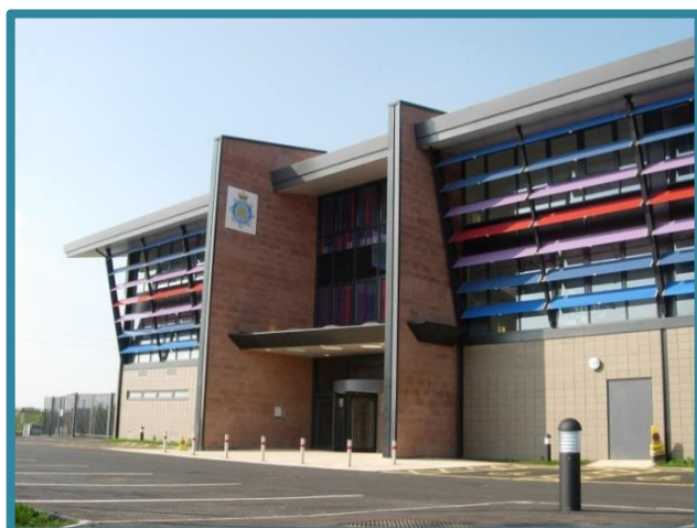
Cumberland BCU HQ – Carlisle
